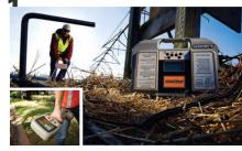
The first responsibility of any excavation or horizontal drilling crew is to locate and mark the location of existing buried pipes, wires, etc. Failure to do so can be costly in terms of damage and fines.....not to mention detrimental to hundreds, if not thousands of people. Failure to accurately locate gas lines and high-voltage power lines can also be harmful or fatal to crewmembers.
